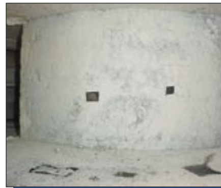
After ten years the fungal wipe samples from the coating surface areas showed an average of 7 cfu/cm2 -meaning nominal growth!
