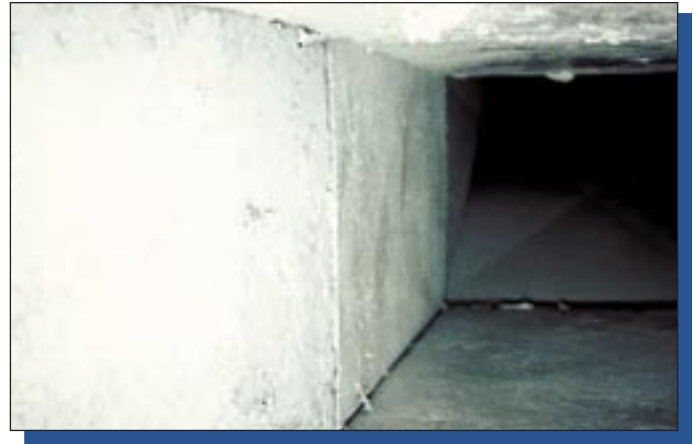
After ten years the fungal wipe samples from the coating surface areas showed an average of 7 cfu/cm2 -meaning nominal growth!
